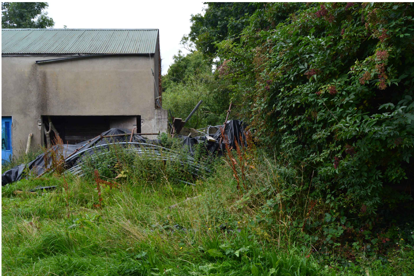
P19: Front Elevation - Two storey Building (Workshop) adjacent to Third Outhouse (No Access)
