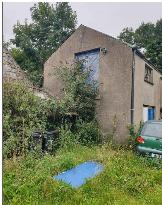
P17: Side Elevation - Two storey Building (Workshop) adjacent to Third Outhouse (No Access)
