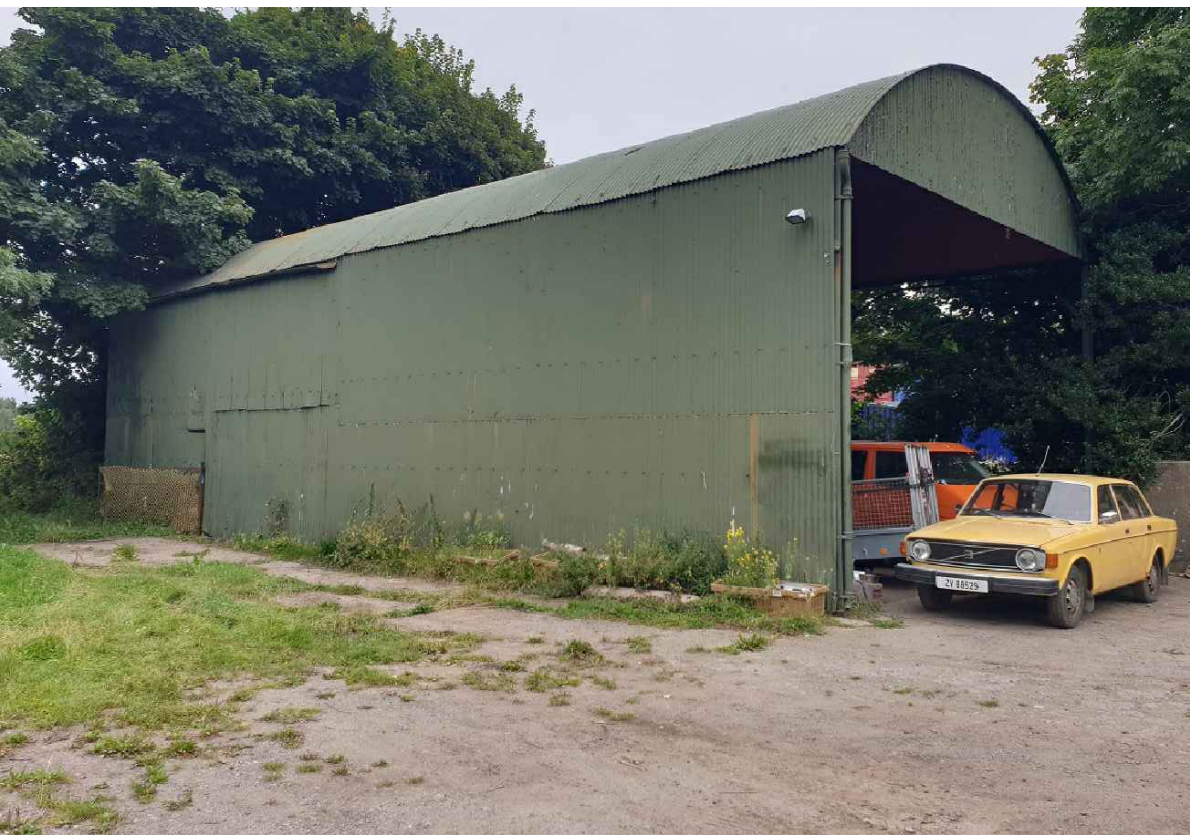
P15: Typical corrugated clad open farm barn NB: Barn to be demolished as part of these works
