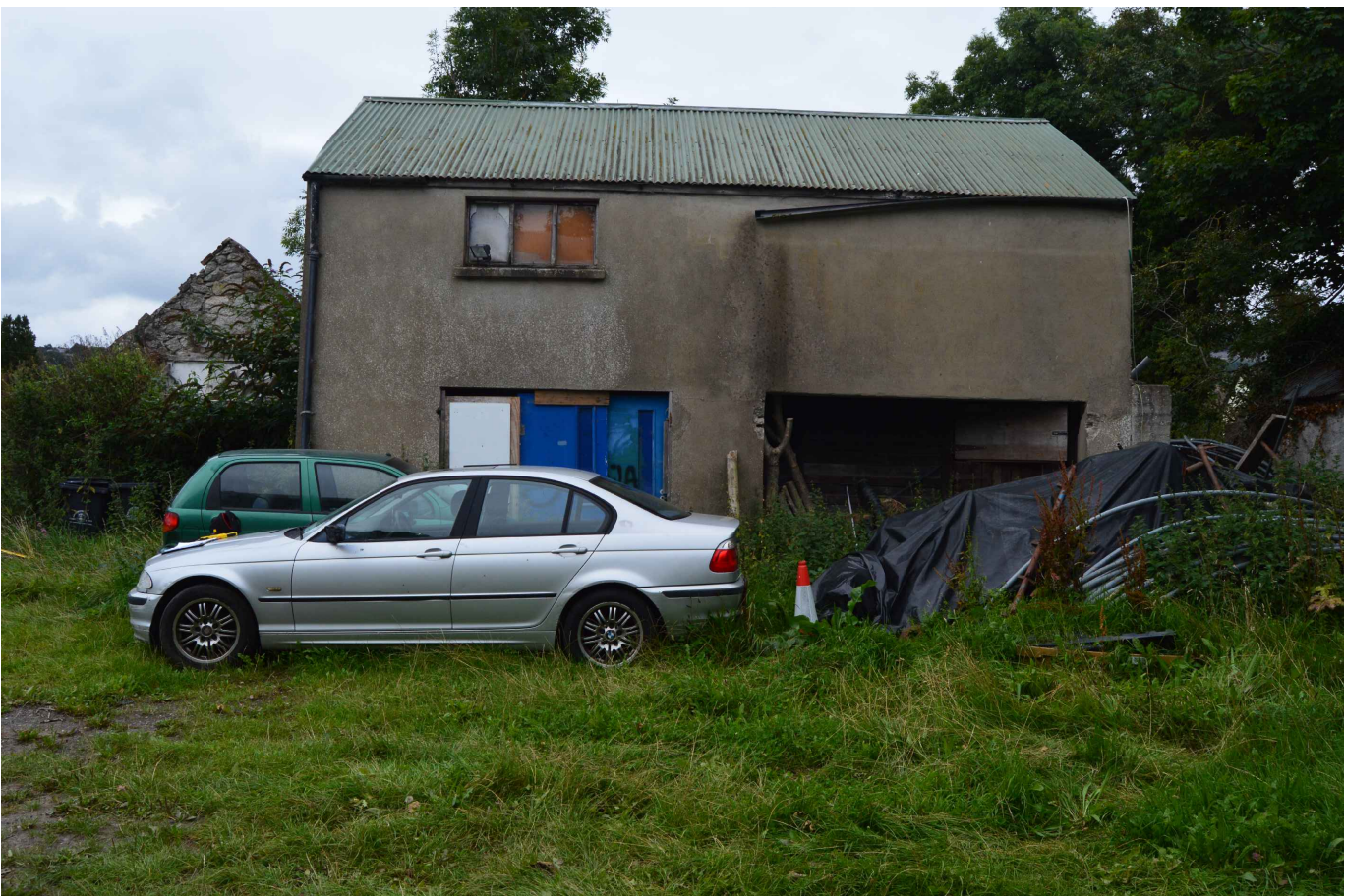
P18: Front Elevation - Two storey Building (Workshop) adjacent to Third Outhouse (No Access)
